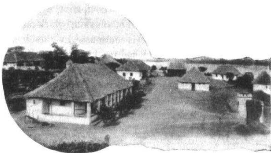
GENERAL VIEW OF BASOKO.
